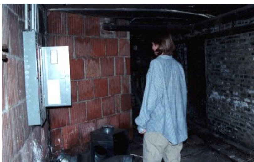
Scott walks around the basement where bodies were once stored. The red firebrick was used to keep down humidity and moisture from affecting the bodies. Picture by Sara Rendall.
